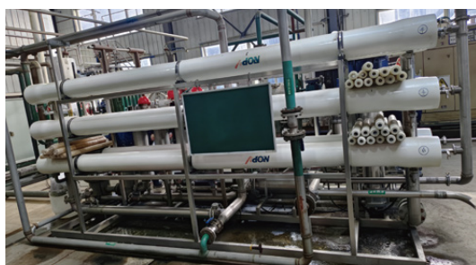
600 tons/day Gibberellic Acid Fermentation Broth NF Unit
